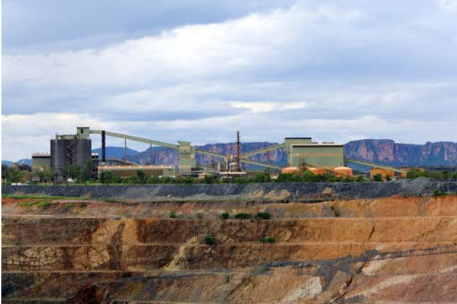
The Ranger plant seen from the open cut pit.
