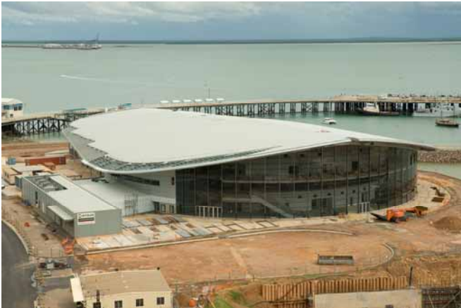
The Darwin Convention Centre under construction at the Waterfront development.
